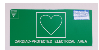
FIGURE 4 Cardiac-Protected Sign Area suitable for CVC insertion provided that the electrical safety test is within date — check the stamp.
